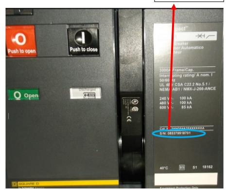
Please refer to safety notice, the list of impacted breakers by serial number is available in the PRB (includes traceability of mechanism block date code AF).
